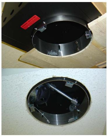
D3. Clean up the magnets and check for proper seating so the cover plate can be held in securely and flush. When finished attach safety cable with screws provided on the ring and panel. SAFETY CABLE MUST BE IN PLACE AT ALL TIMES TO PREVENT POSSIBLE SERIOUS INJURIES OR PROPERTY DAMAGE DUE TO FALLING COVER PLATE!
